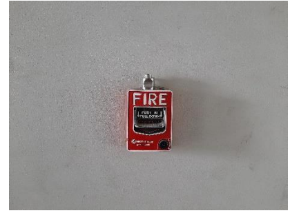
fire alarm manual station
